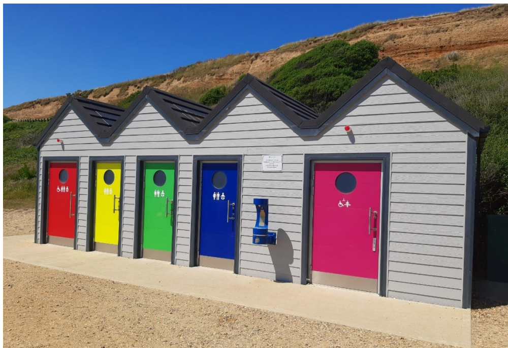
Barton Beach Public Toilets
